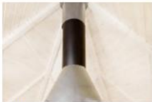
Grill Chimney Extension
