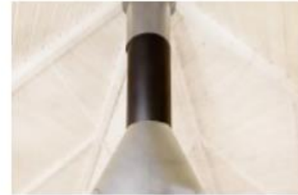
Grill Chimney Extension
