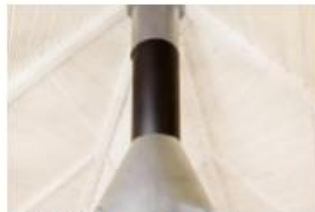
Grill Chimney Extension
