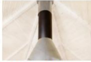
Grill Chimney Extension
